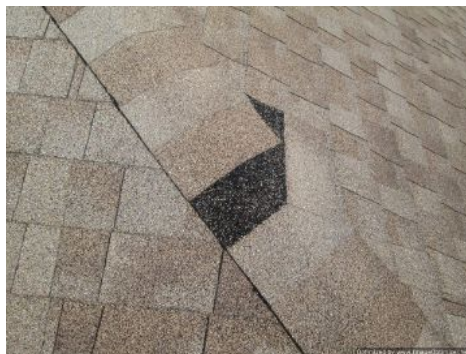
Damaged Shingle
