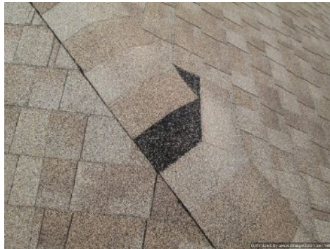
Damaged Shingle
